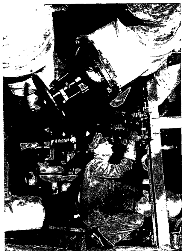
Plant engineer checks control valve in campus 3-mile underground tunnel system.
