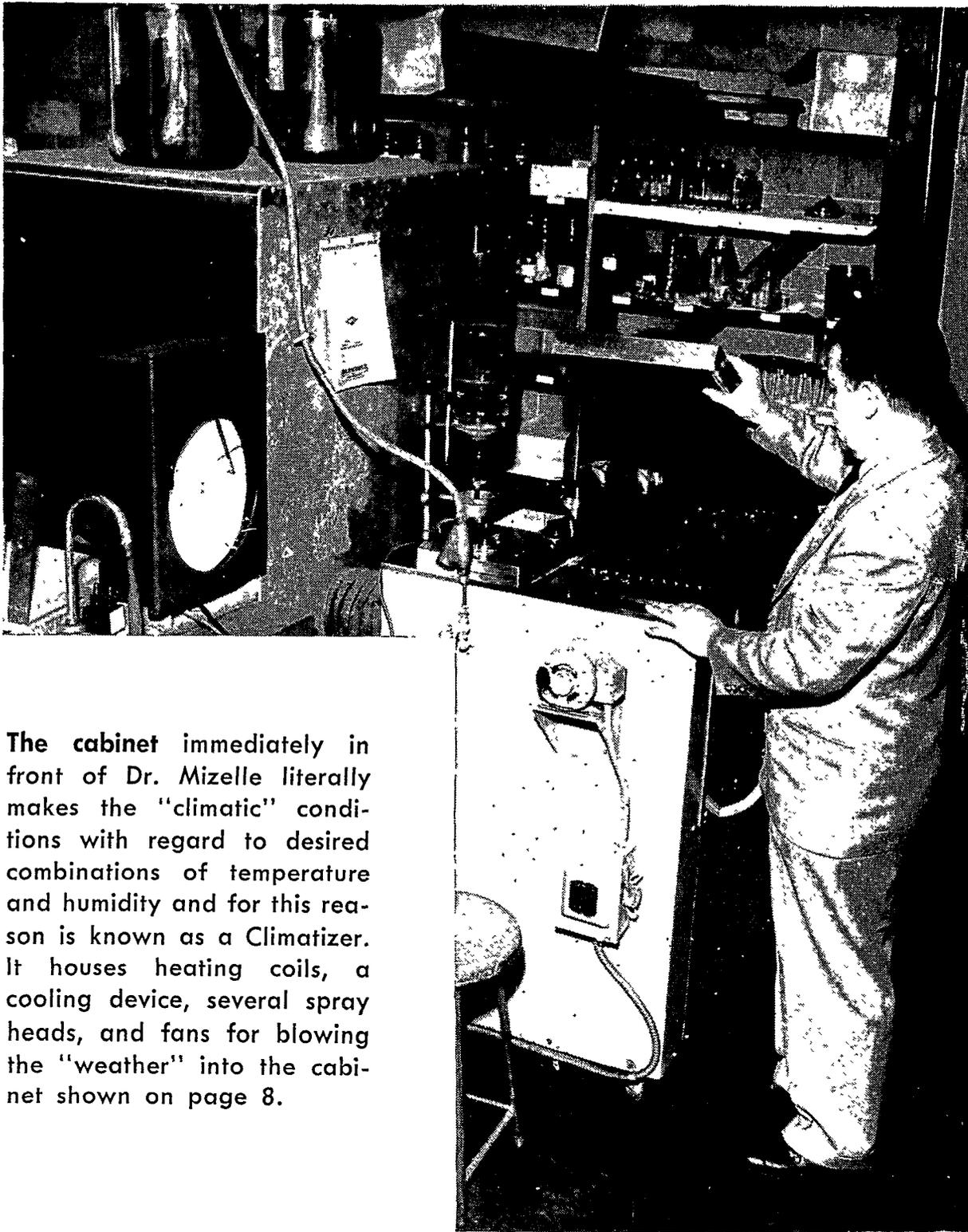
The cabinet immediately in front of Dr. Mizelle literally makes the "climatic" conditions with regard to desired combinations of temperature and humidity and for this reason is known as a Climatizer. It houses heating coils, a cooling device, several spray heads, and fans for blowing the "weather" into the cabinet shown on page 8.
