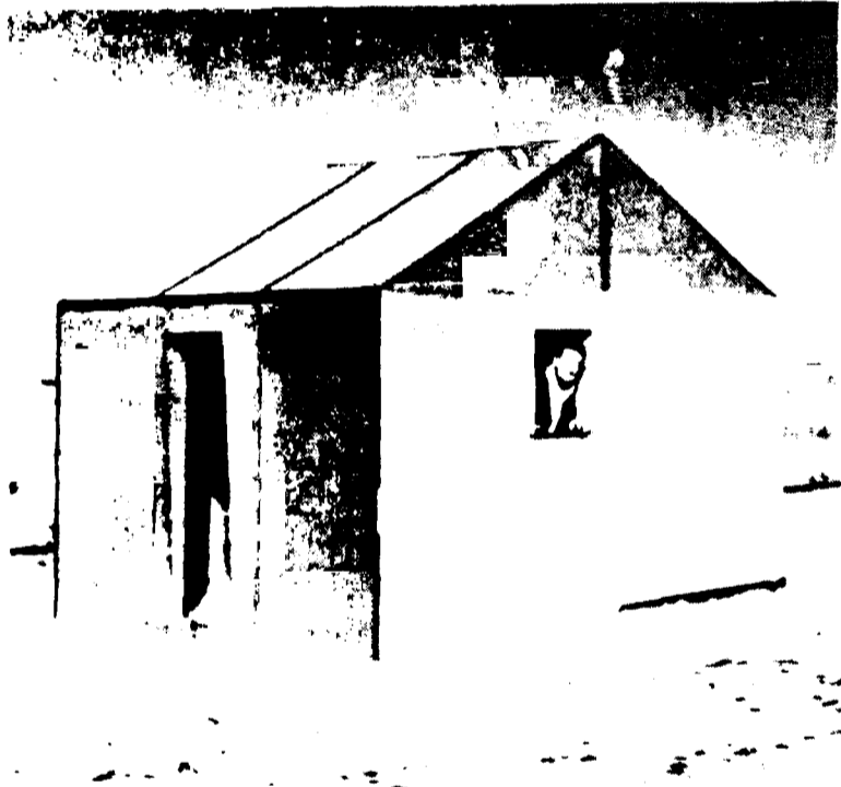
Notre Dame students and alumni journey to Guatemala over break to test corrugated fiberboard structures. The cardboard was used to erect temporary shelter for victims of the recent Guatemala earthquake.
