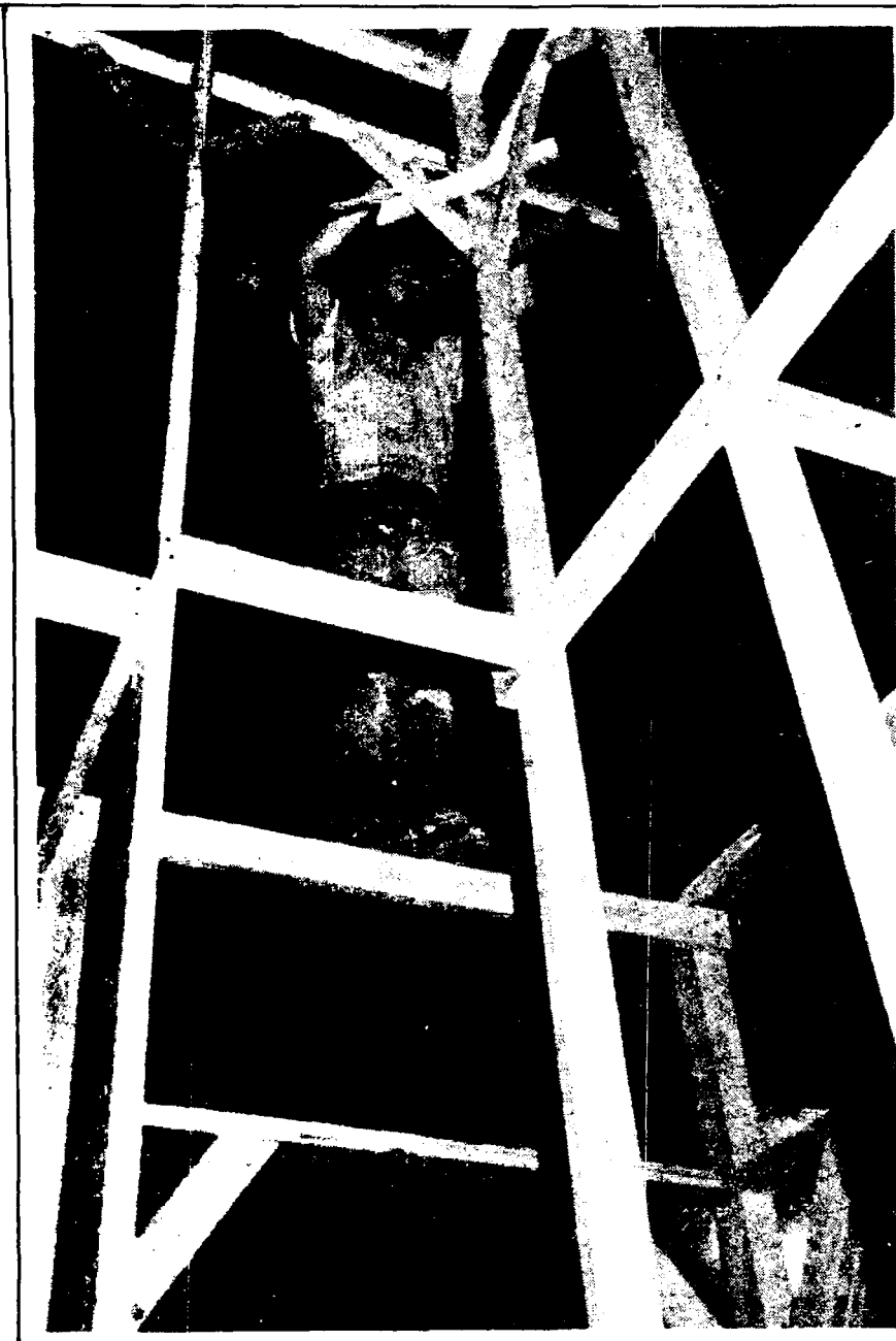
Mardi Gras booth construction has begun, turning Stepan Center into a builder's workshop. The theme of Mardi Gras 1978 is "Expo N.D." Construction will continue until Feb. 3. The dealers will then man the booths until Feb. 12. [Photo by Ron Szot.]
