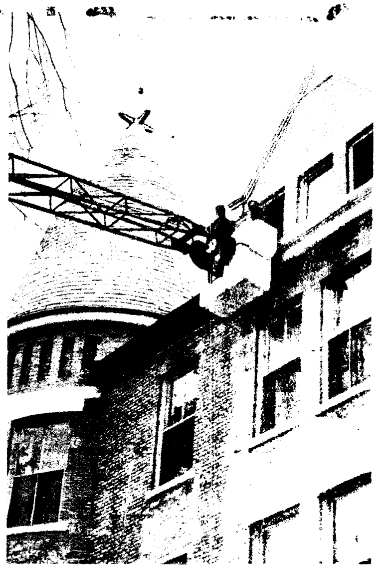
Workmen yesterday began spring repairs on the gutter of Sorin Hall. Will the potholes on Ho-Chi-Min be fixed next? [Photo by Ken McAlpine]
