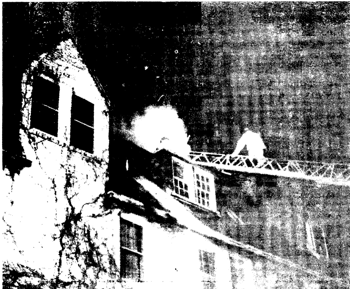
Firemen climb to the top floor of Howard Hall to fight the blaze which reportedly began early this morning in an elevator shaft. [Photo by Ken McAlpine]
