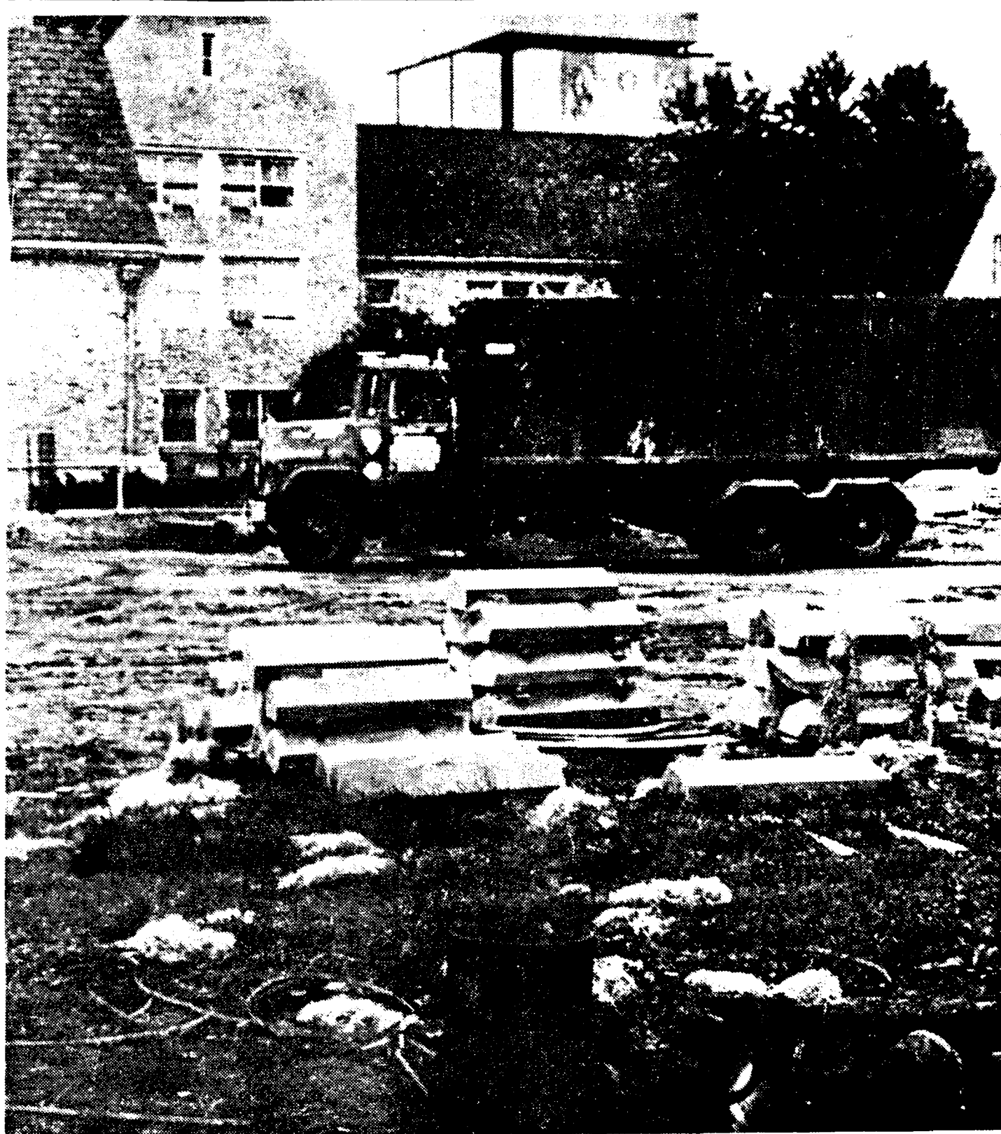
Construction continues on the Engineering Annex, leaving its mark upon the O'Shag grounds. [Photo by Mark Ricca]
