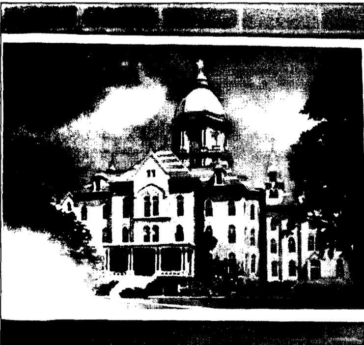
This Golden Dome post card was commissioned in 1992, part of a historical buildings commemorative series offered by the Postal Service.
