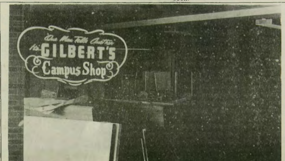
The old Gilbert's campus store is now undergoing renovation and will become an extension of the bookstore. Bro. Conen Moran, bookstore manager, says
