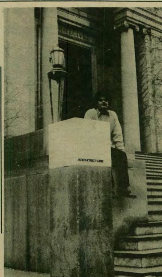
A new lighting fixture, above right, designed to be placed at major entrances of campus buildings, has been unveiled for review by the Campus Planning department of the School of Architecture. The fixture, composed of an aggregate concrete formwork and plexiglas head, is proposed to improve campus lighting and to assist in finding the location of University buildings. Dom Carbone, pictured above, engineered the project. A Keenan Hall resident has obviously foreseen this as a problem and has created his own temporary solution, above left. Comments and questions are invited and should be addressed to Esmee Bellalta, Department of Architecture. [Photos courtesy Department of Architecture]
