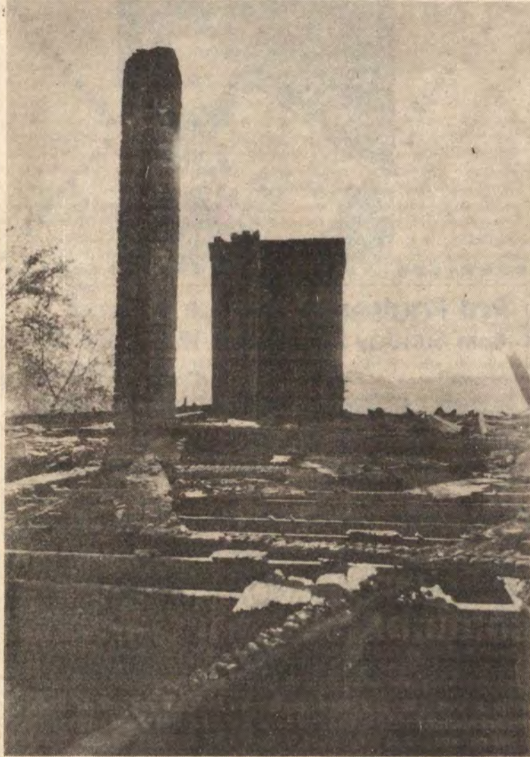
Arson partially destroyed the ND boathouse on Oct. 23. Investigators are continuing the search for the suspect. [photo by Greg Solman]
