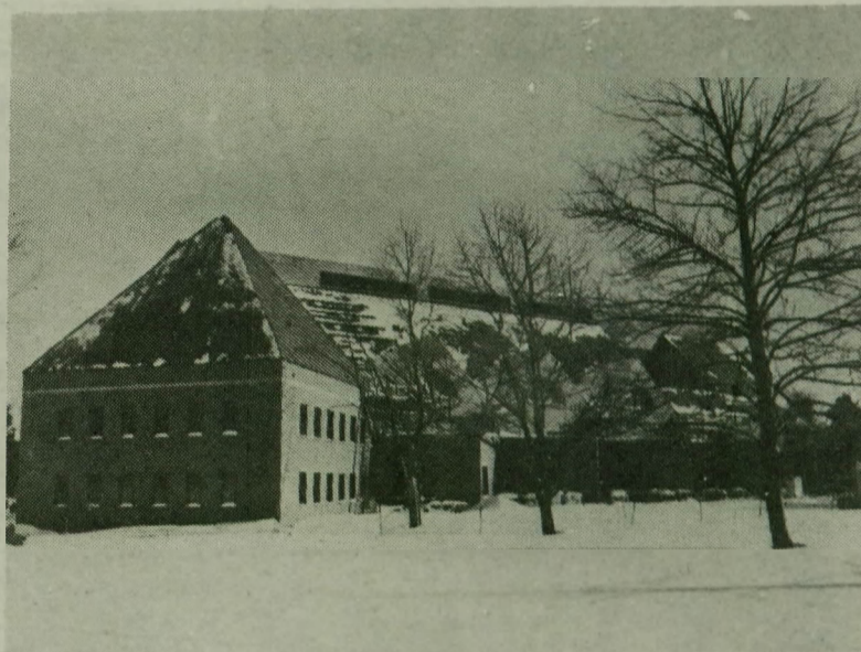
The construction of St. Mary's new library continues through the winter, and the completion of the facility is near at hand. (Photo by John Macor)
