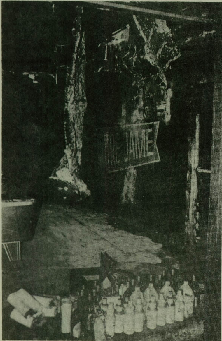
Corby's Tavern was gutted by a fire last Sunday morning. The fire, which started in a furnace, extensively damaged the interior of the establishment. See accompanying story. (Photo by John Macor)
