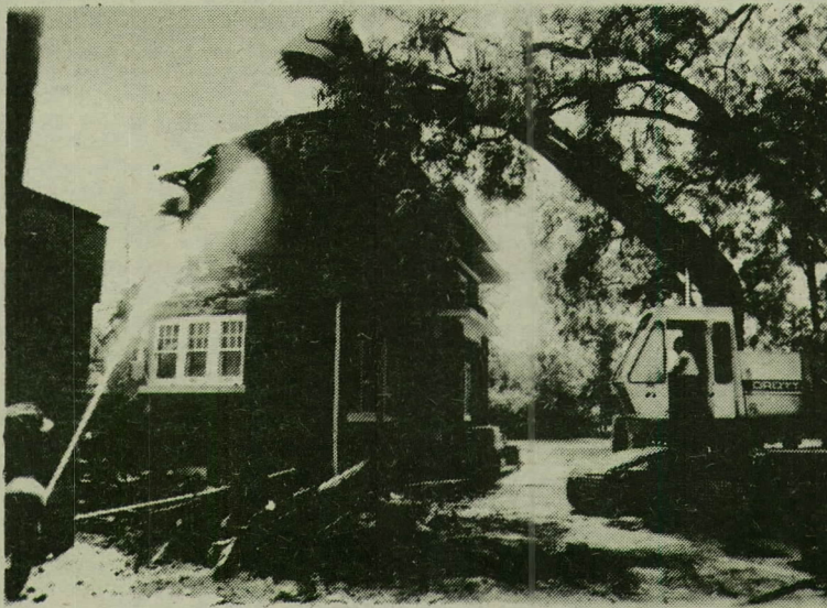
Workers use a crane and fire hoses to demolish the old Senior-Alumni Club. The new club can be seen on the left. See story at left. (Photo by Scott Bower)
