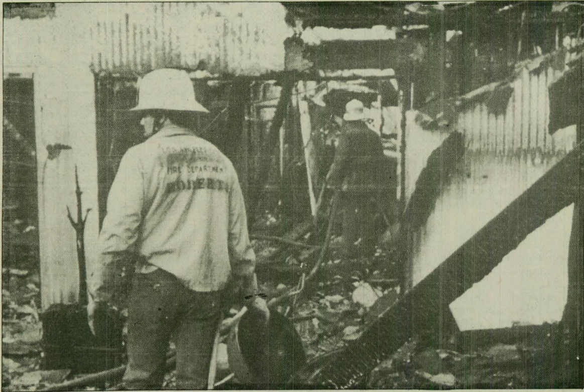
These are the remains of the Los Angeles home of Laker star Kareem Abdul-Jabbar. The house was gutted by a fire early Monday morning that
