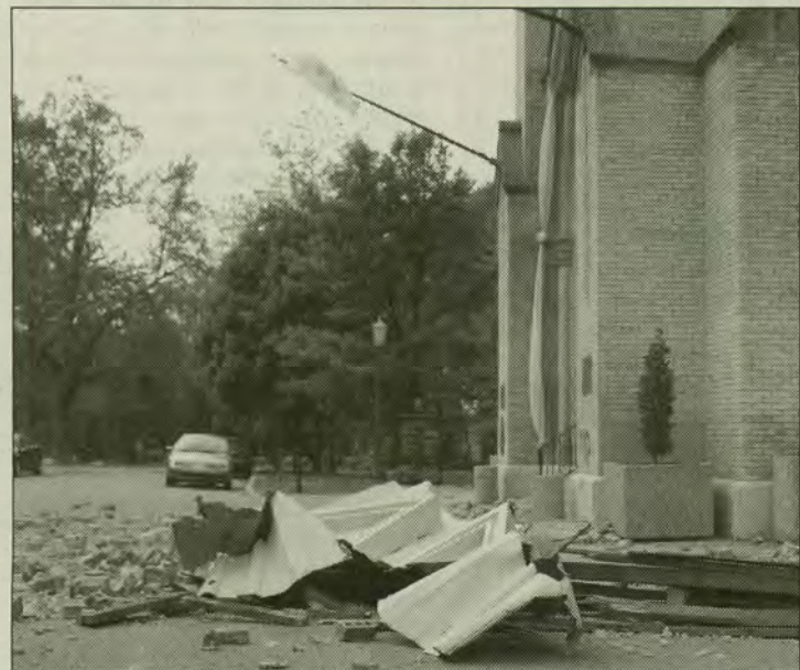
CHRISTIAN SAGARDIA/The Observer Wreckage from a spire on top of the Basilica lays in front of the building after strong winds caused it to fall Tuesday.
