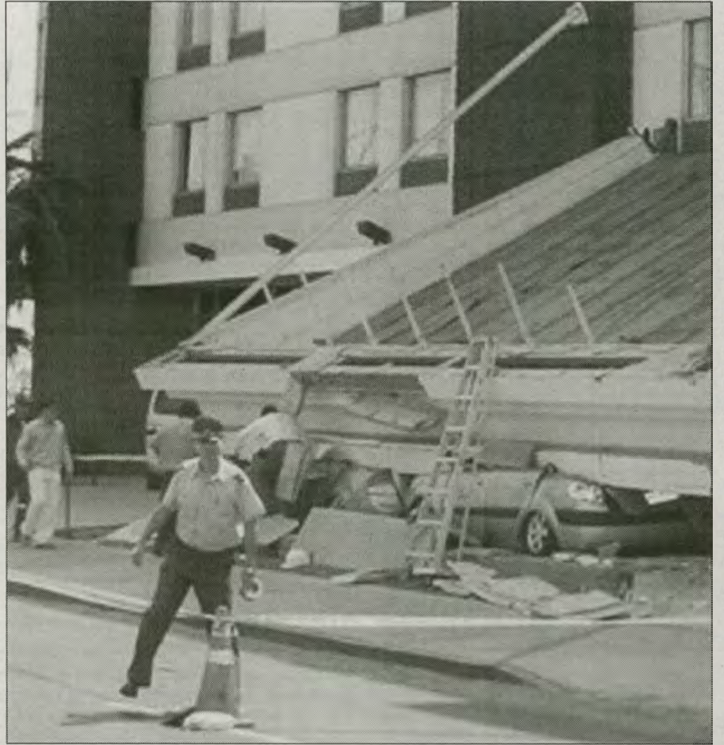
Officials rope off a scene that resulted from Wednesday's 7.7 earthquake in northern Chile where several cars were crushed after a roof collapsed.
