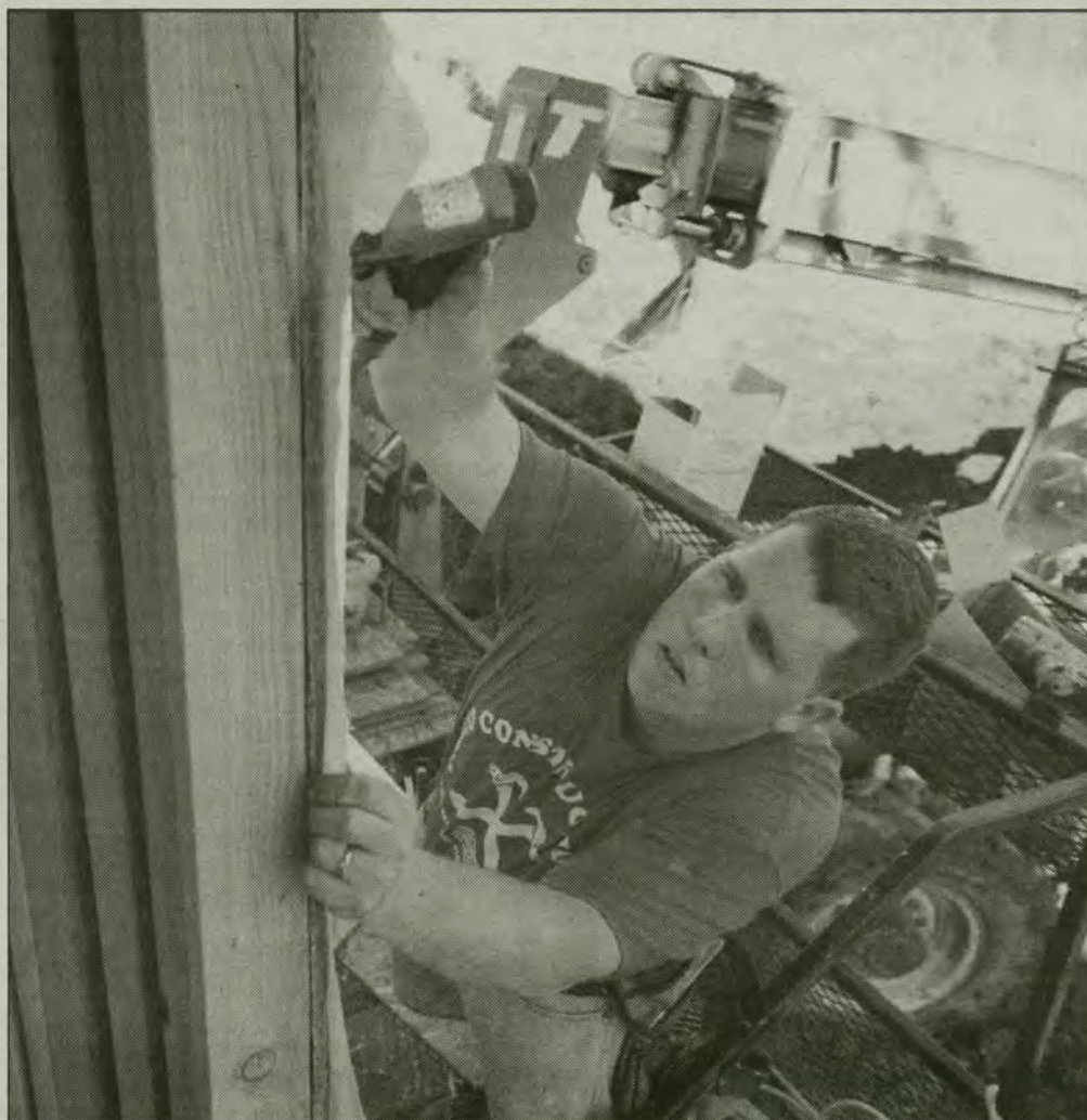
A new house is under construction in Iowa. The Department of Commerce reported that housing construction increased by 22 percent in February.
