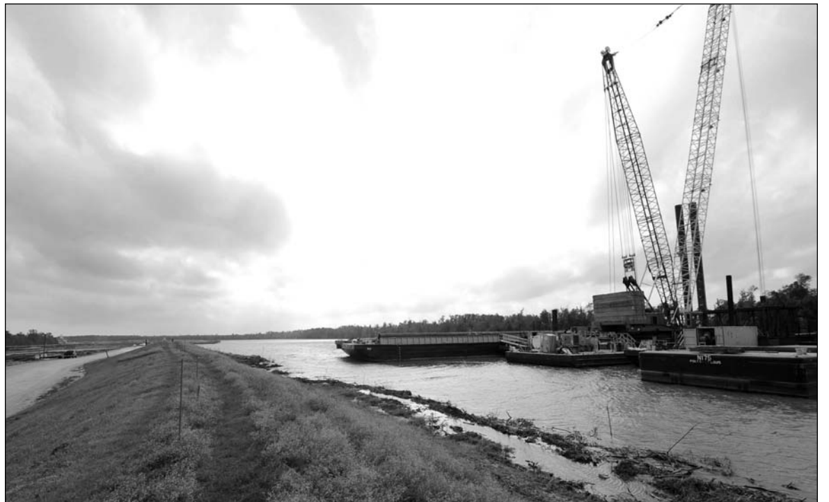
In an Oct. 30 file photo, the West Closure Structure project in Harvey, La. is shown. When finished, the structure will close off navigation and drainage canals that turn into conduits for storm surge during hurricanes.
