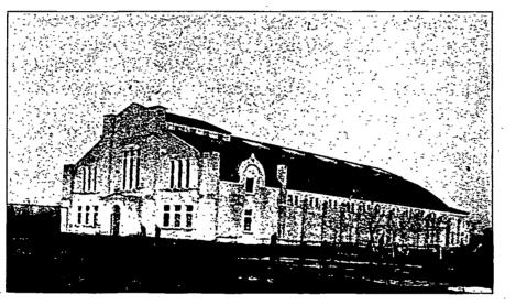
important consideration in the building of the gymnasium. The room is 169 x 100 feet with walls 25-feet high. The roof is supported by semicircular iron trusses, ten in number, which rest upon the side walls. Light is admitted through
