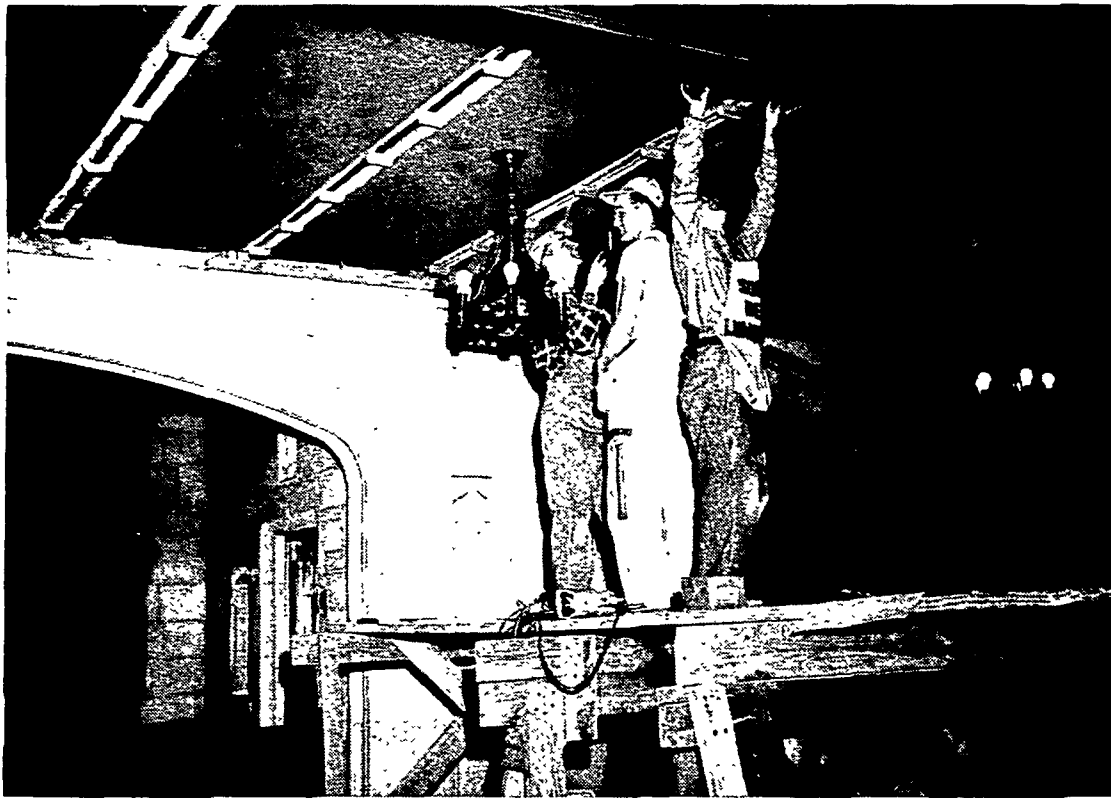
DILLON HALL CHAPED REPAIRS — Three men on a Horse (Wooden)
