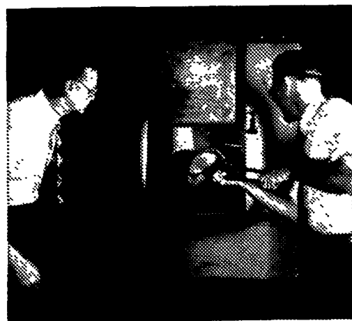
C. M. Olson, Ph.D.Phys.Ch., Chicago '36, and C. H. Winter, Jr., B.S.Ch.E., Virginia Polytechnic Institute '40, removing 100-lb. titanium ingot from furnace in heat-treating study.
