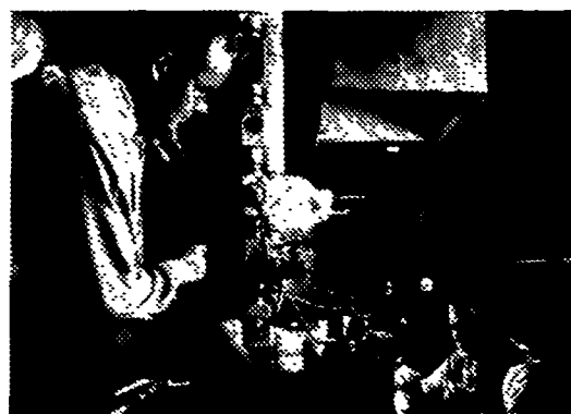
Uniquely designed adapter for a screw extruder under study by Ralph J. Covell, B.S.M.E., Purdue '49, and John F. Bowling, B.S.M.E., Purdue '41. The adapter heats, filters and forms polymer into filaments.
