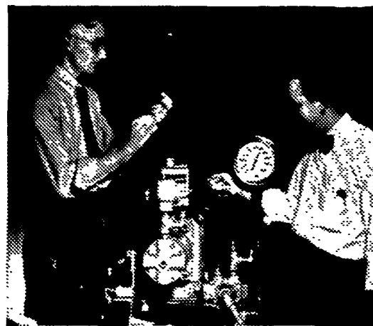
Ralph C. Grubb, B.S.M.E., Tennessee '51, and Paul D. Kohl, B.S.M.E., Purdue '46, study characteristics of a super-pressure pump (75,000 p.s.i.) designed by Du Pont engineers and made in Du Pont shops.
