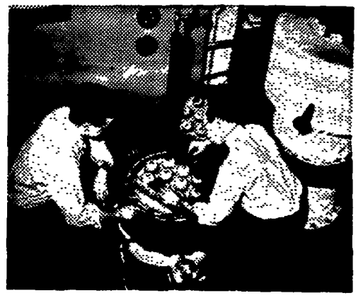
STUDYING plate in stainless-steel tower used to determine efficiency of designs: C. M. Gamel, Jr., S.M.Ch.E., M.I.T. '48; and J. B. Jones, M.S.Ch.E., University of Michigan '46.
