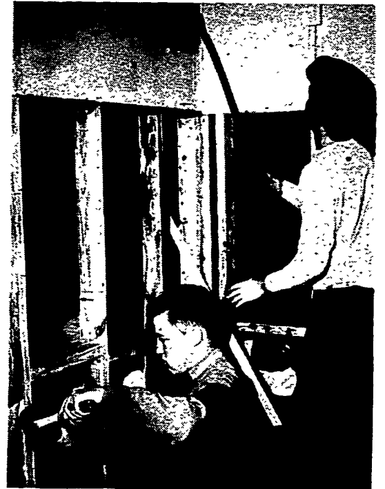
CENTER CROWBAR CREW Constructive Destruction
