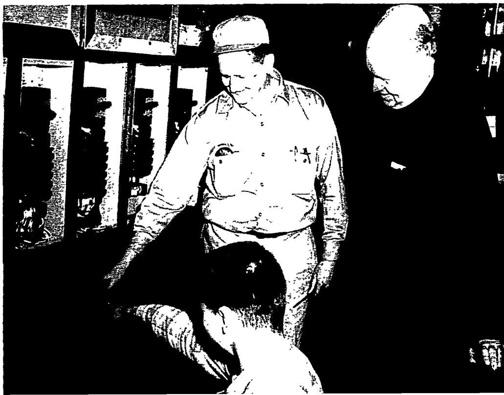
Maze of switches on the new lighting control board.
