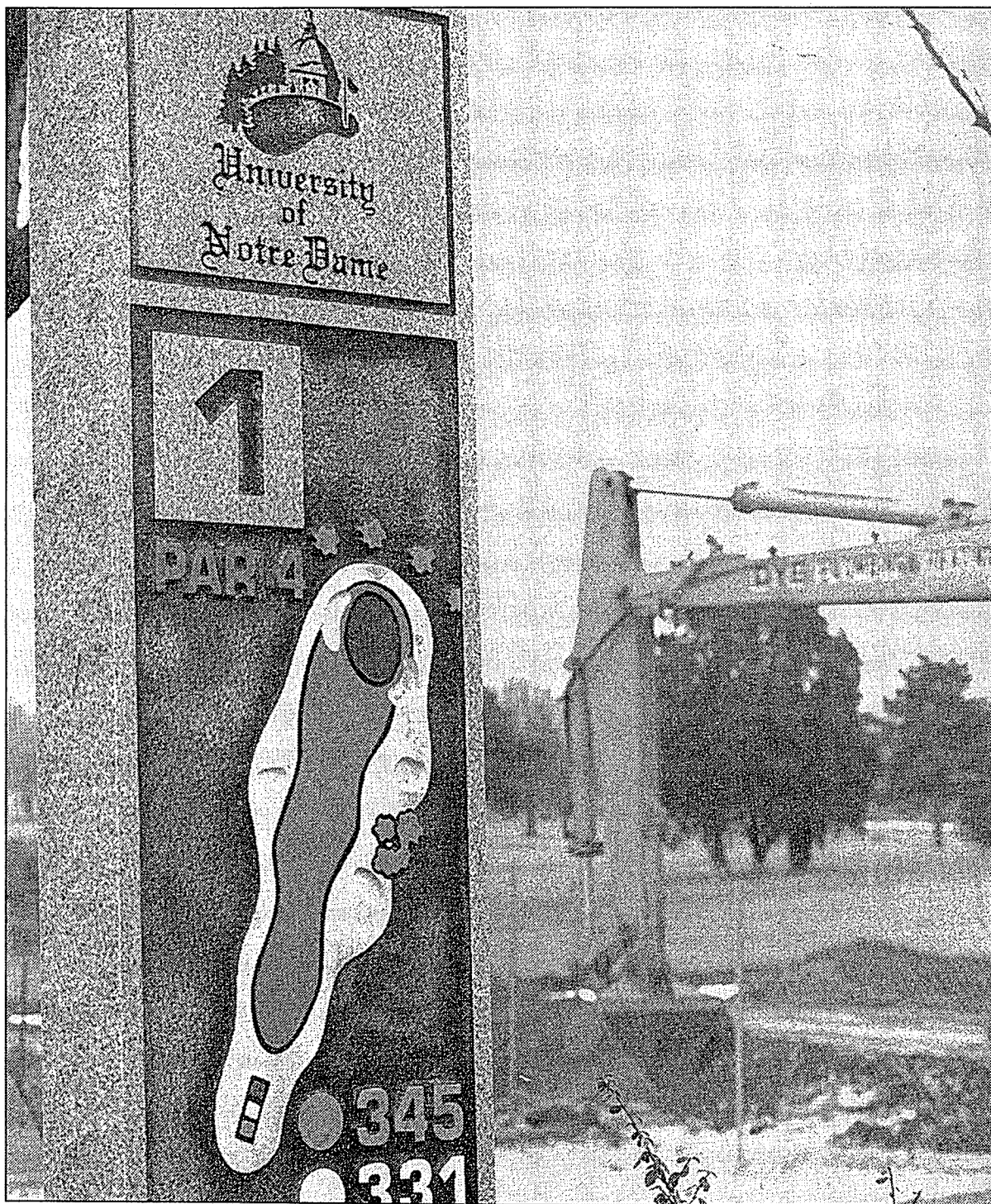
Making way for the two new South Quad dorms, construction equipment tears up the Burke Memorial Golf Course.
