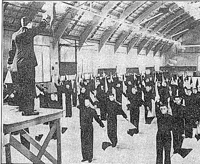
Semaphore class is conducted for NROTC students and Midshipmen candidates in the Navy Drill Hall, which the university constructed for military training during World War II. The Navy Drill Hall, which used to lie behind the old Fieldhouse, was demolished after the war, but the "Middy School" building, which provided classroom and office space for NROTC and the Midshipmen's school, is currently the headquarters for campus security.
