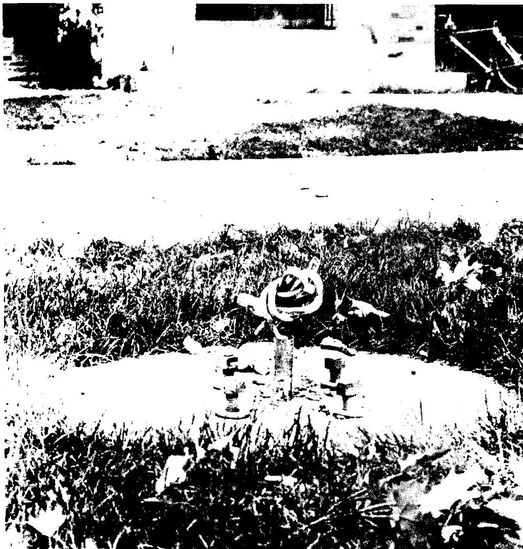
AND THEN THERE WAS DARKNESS!!! The concrete foundations used for the light fixtures on the North Quad have made for at least two safety hazards: the darkness and tripping over the bases in the dark.
