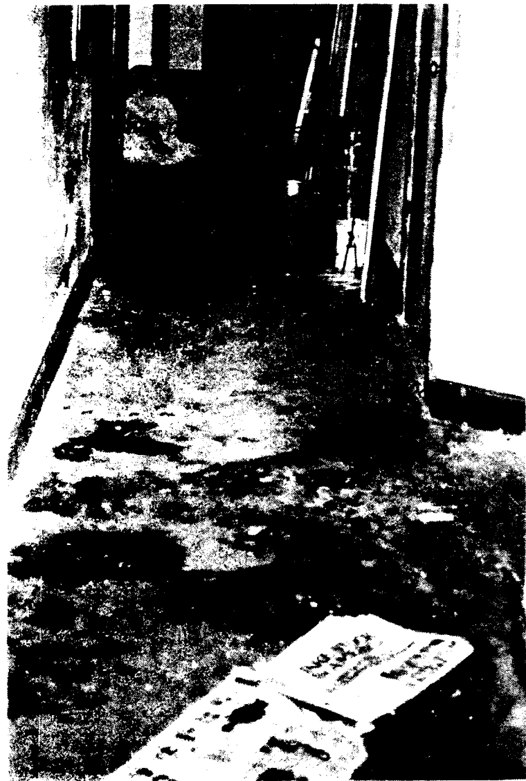
Waterspots stain the floor in this Howard hallway as a result of the fire which occurred March 16. Most of the hall has been restored to normal, however. [Photo by Bill Reifsteck]
