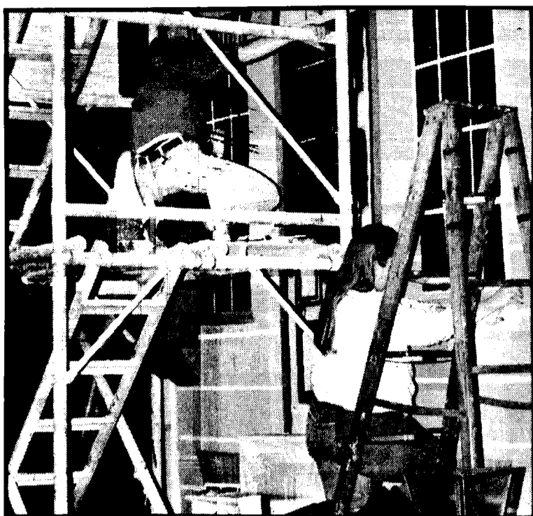
Construction crews diligently prepare for the festivities of Mardi Gras. [photo by Tracy Jane McAuliffe]
