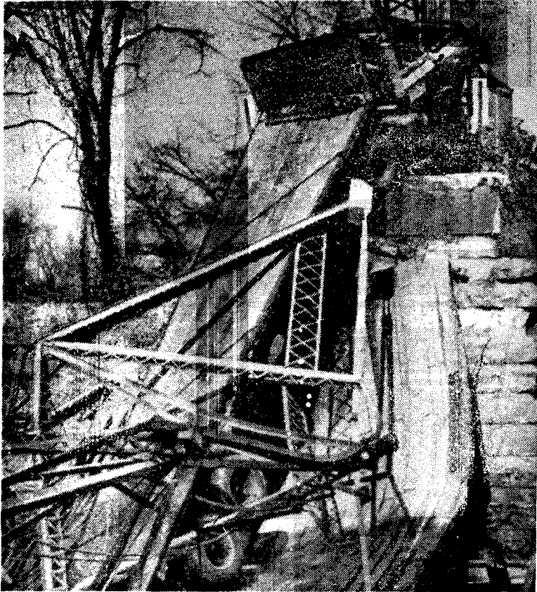
The driver of this Akron, Ohio semi-trailer truck walked away without a scratch after a bridge over Cole Creek, near Veedersburg, Ind., collapsed under the weight of 117,000 pounds of steel the truck was hauling. Police said the truck was at least 57 tons too heavy for the old structure, on Indiana 32 in Fountain County. (AP Laserphoto).
