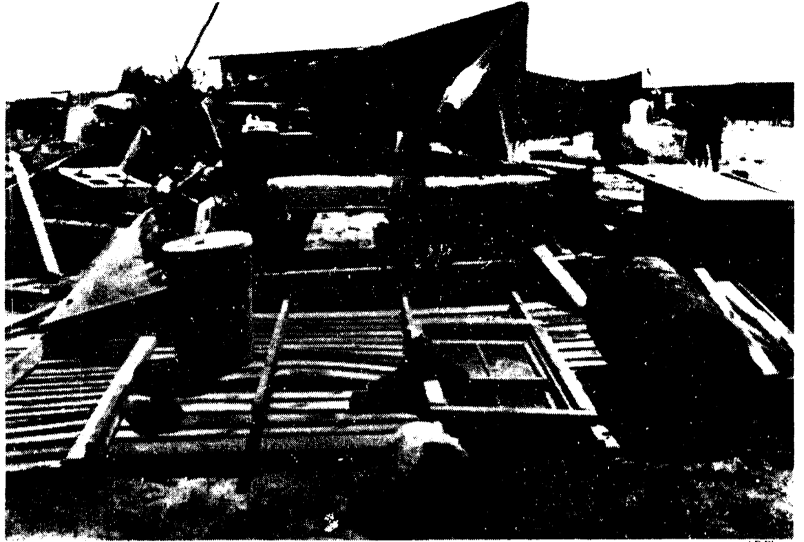
A home in the fishing village of LaMedia Luna, Mexico was completely destroyed by the force of hurricane Barry. This small remote fishing town
