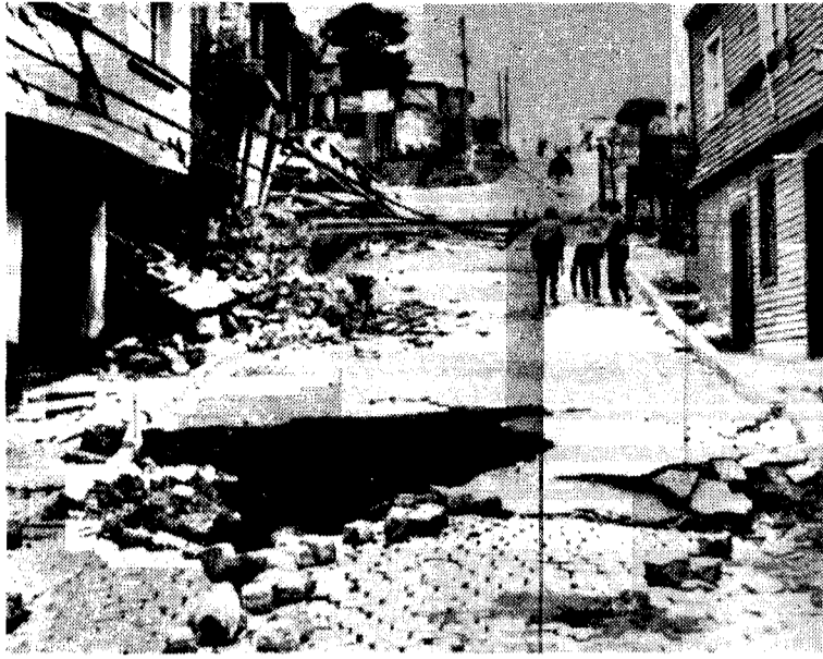
This street in San Antonio near Santiago de Chile was completely destroyed after a massive earthquake shook central Chile Sunday night.
