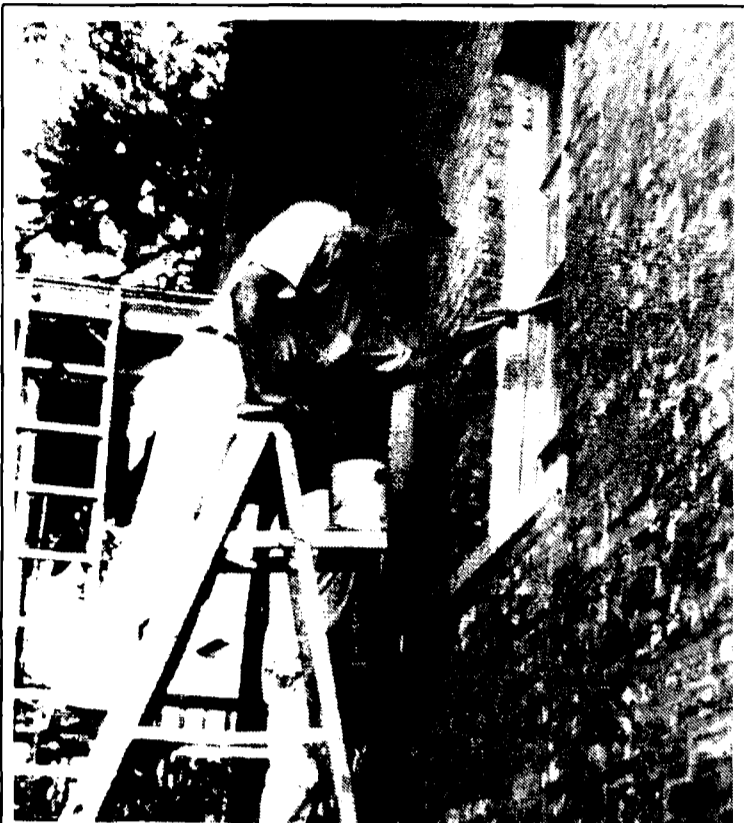
Preparing Old College The Observer/John T. Rock Workers paint Old College getting ready for the sesquicentennial celebration. Old College is the first and oldest building on campus, built in the spring of 1843.
