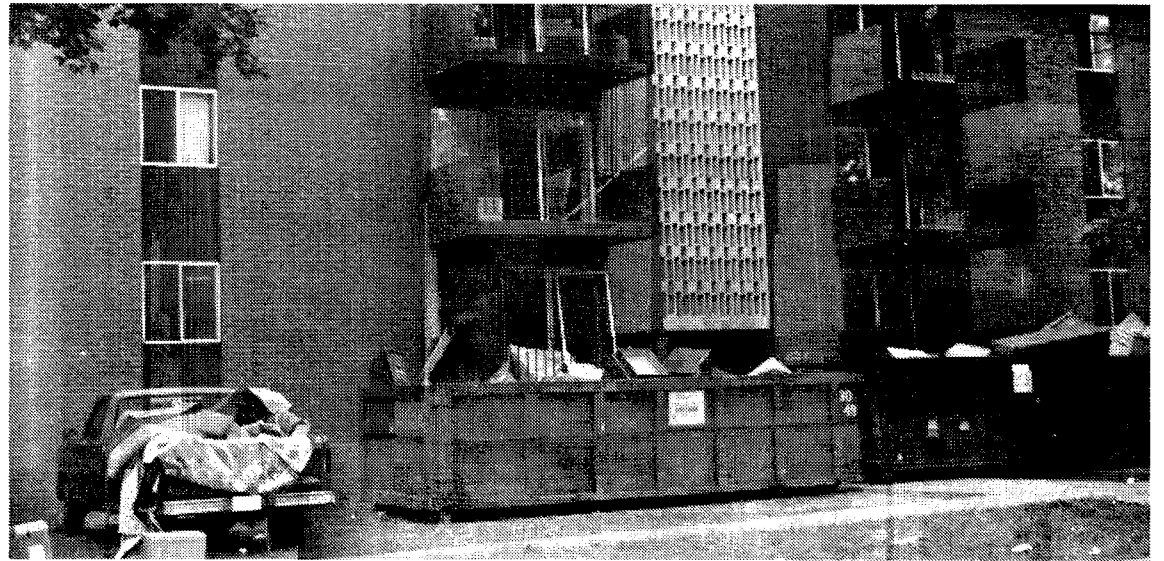
The Observer/Marguerite Schropp Notre Dame Ave. Apartments have been bought by the Northeast Development Company and will be open to student residents in the spring.
