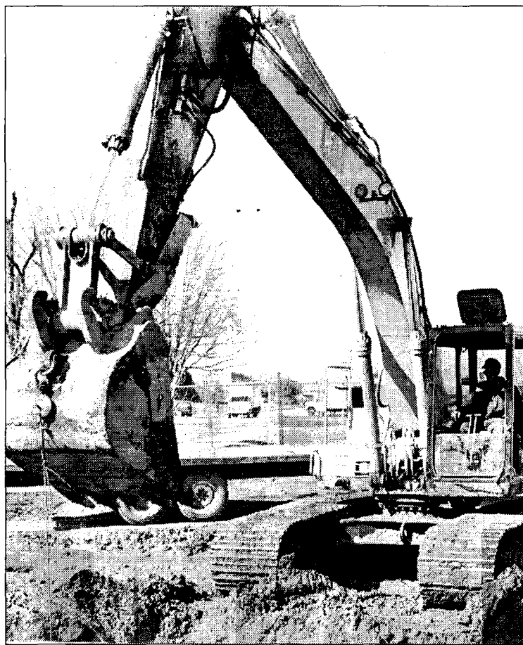
The Observer/Bret Hogan The installation of new water lines under the Stepan courts should be done in time for Bookstore Basketball.
