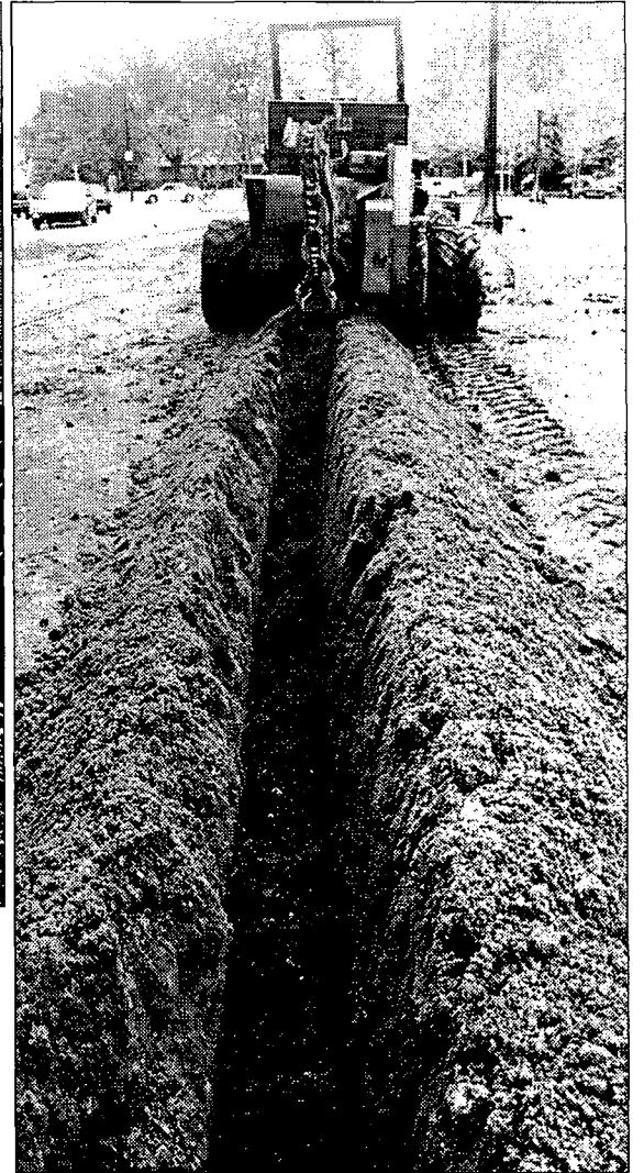
Tractors dug trenches as part of the new stadium's underground sprinkler system.
