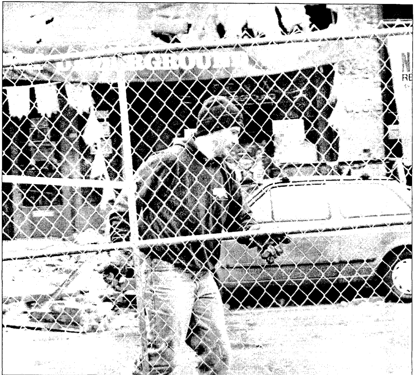
An unidentified worker constructs a fence in front of a popular night spot in downtown Seattle which was closed after a large part of its facade fell during a magnitude 6.8 earthquake. Seattle is still addressing the damage. KRT Photo
