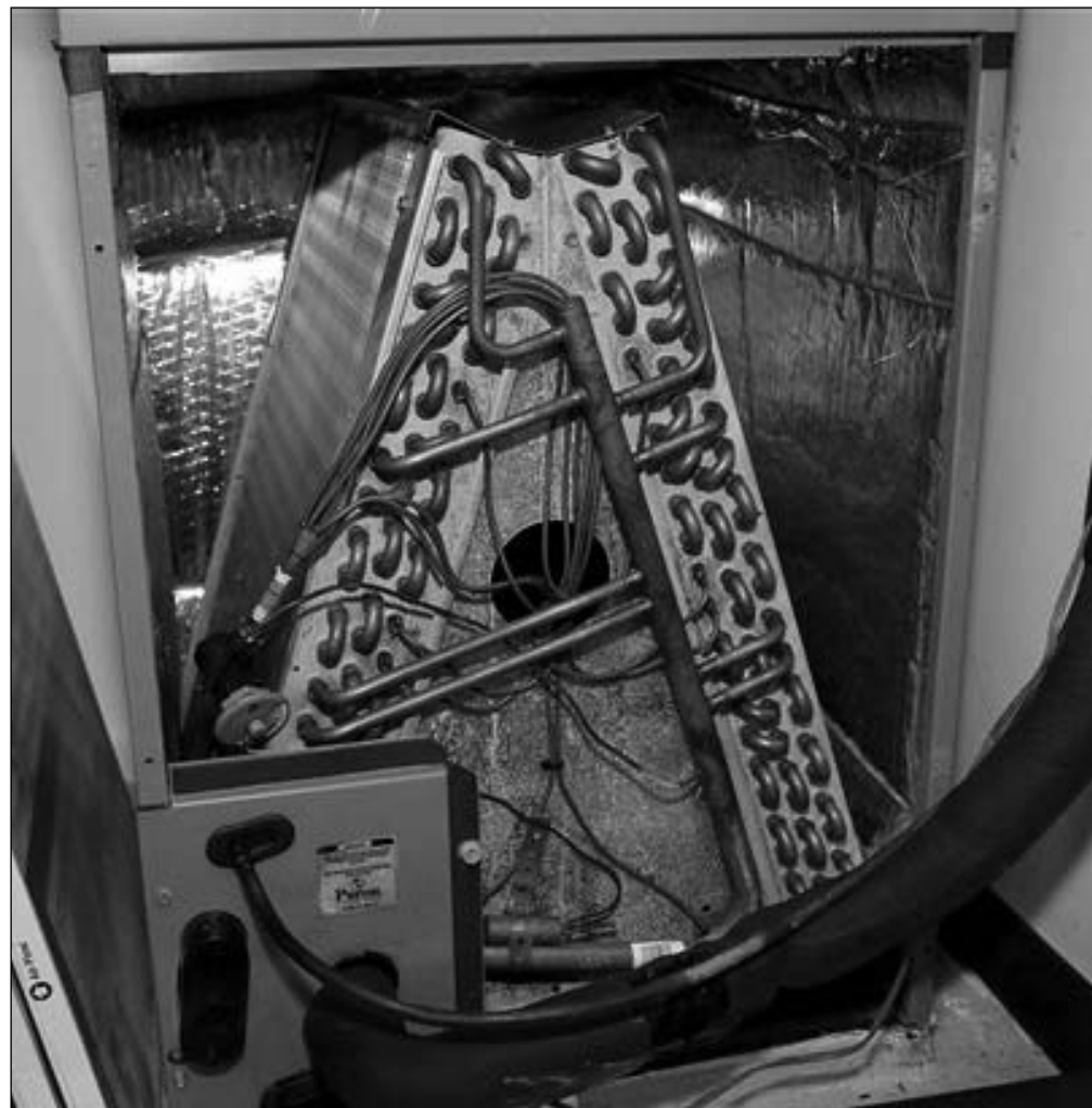
An air conditioner coil shows some corrosion because of contact with Chinese-made drywall in the home of James and Maria Ivory in Punta Gorda, Fla.
