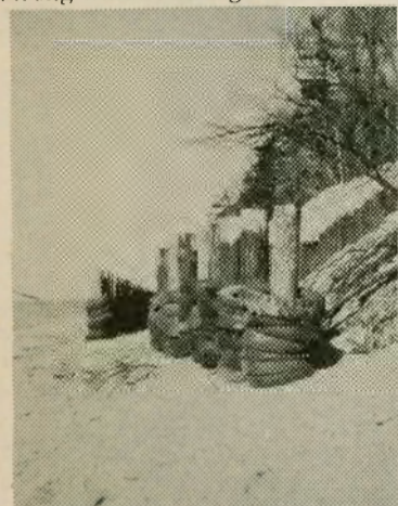
In areas the beach has been almost entirely eroded.
