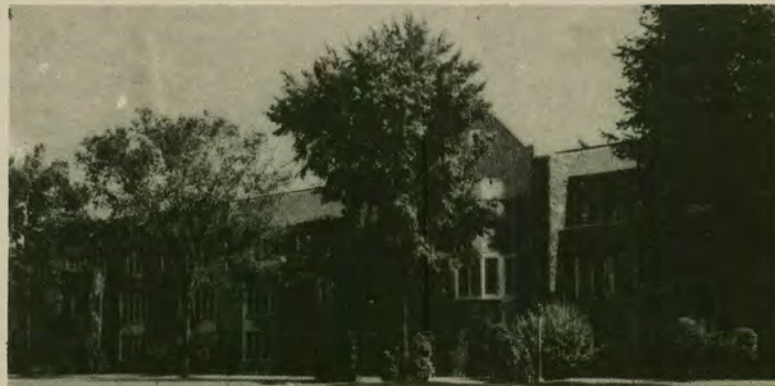
CUSHING HALL of Engineering's expansion program will not begin for at least three months. The long range plan is to eventually house all departments and labs in one complex.
