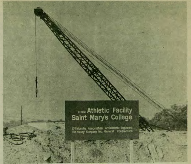
Construction is under way on St. Mary's new athletic complex. The building is scheduled to be completed by next March.
