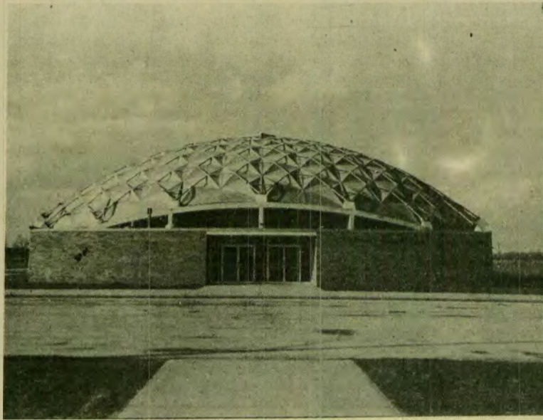
No, that's not a futuristic building on Mars, that's Stepan Center (photo by Debbie Krilich)
