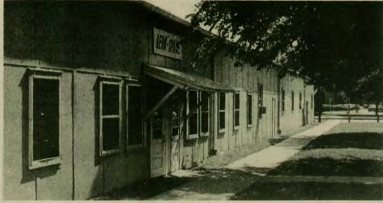
The Aero-space building [Photo by Greg Trzupek]
