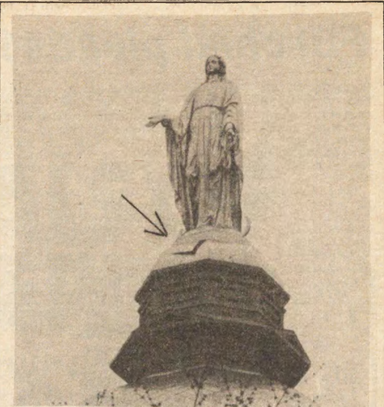
Due to the winter winds and weather, six doors situated at the base of the statue of Our Lady on top of the Golden Dome worked themselves loose. The doors have been rechained and secured, Maintenance said. [Photo by Sue Coliton]
