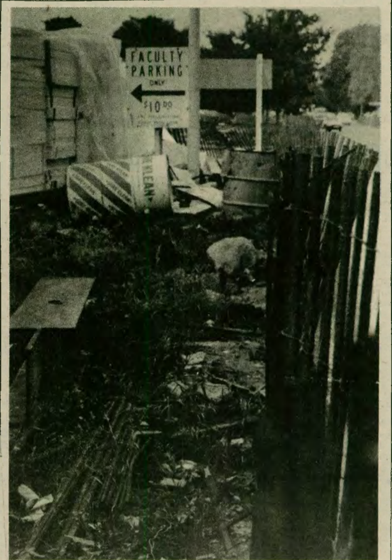
General rubbish and refuse clutter the side lawn of O'Shag as the construction continues on the Engineering Building. [Photo by Mark Ricca]
