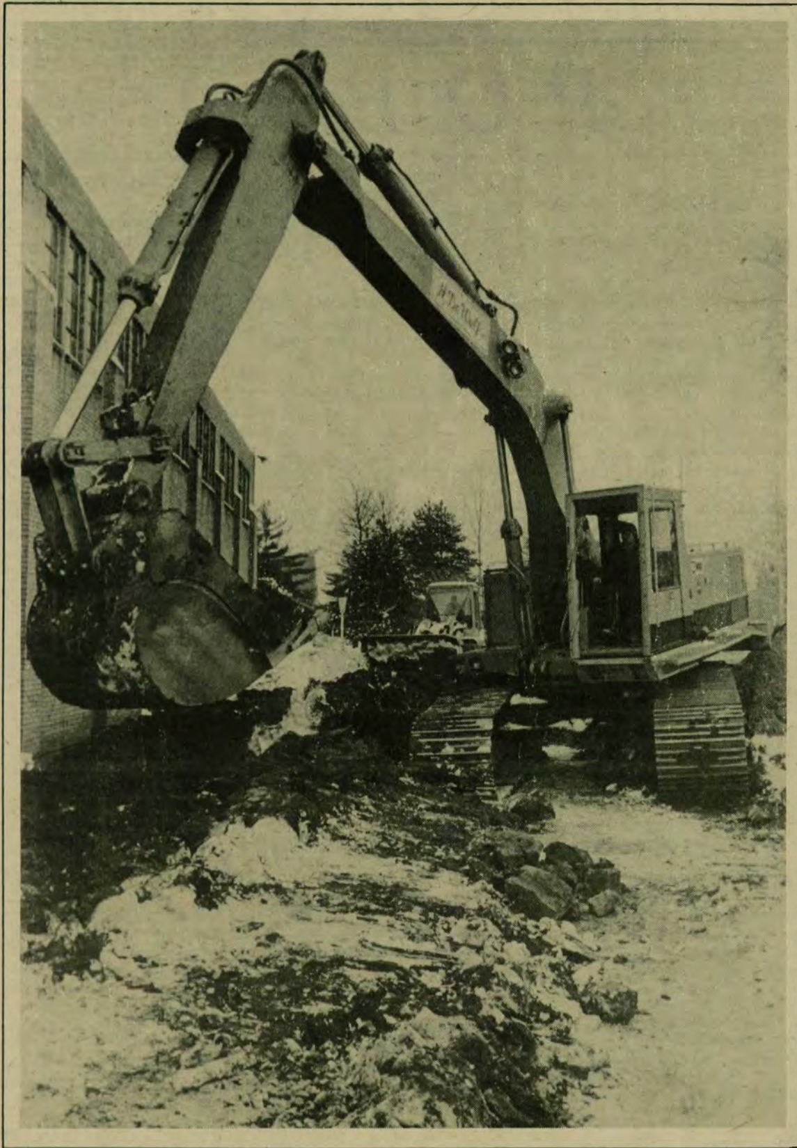
Plumbing repairs near the fieldhouse obstructed student walkways on the first day of class yesterday. [Photo by Dave Rumbach]
