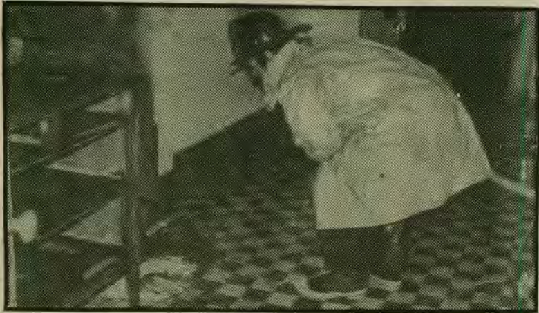
Fireman inspects damage at Augusta Hall. Story begins on page 1 and is continued below. [Photo by Phillip Johnson]
