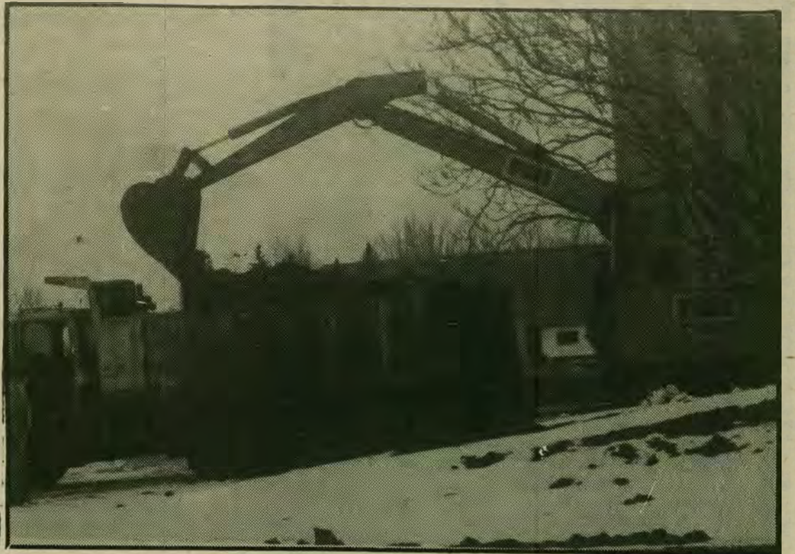
Construction continues on the new dorms near the library. [photo by Tom Jackman]
