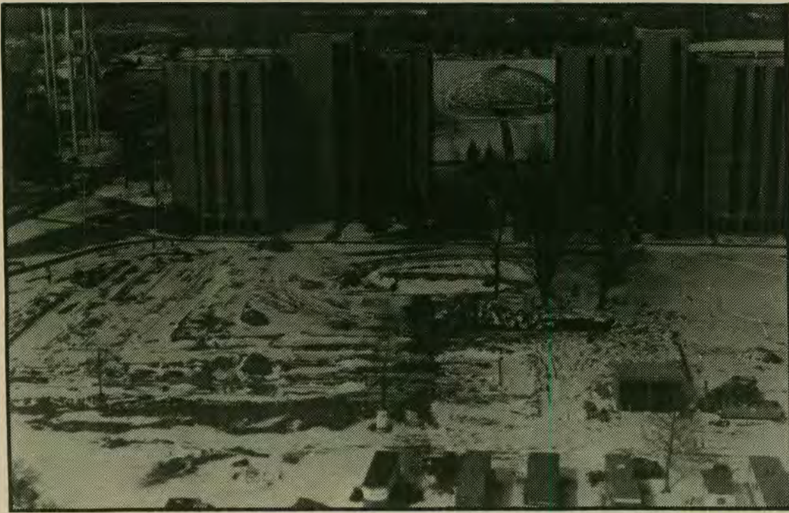
Recent snowstorms have delayed construction on the new dorms. [photo by John Macor]
