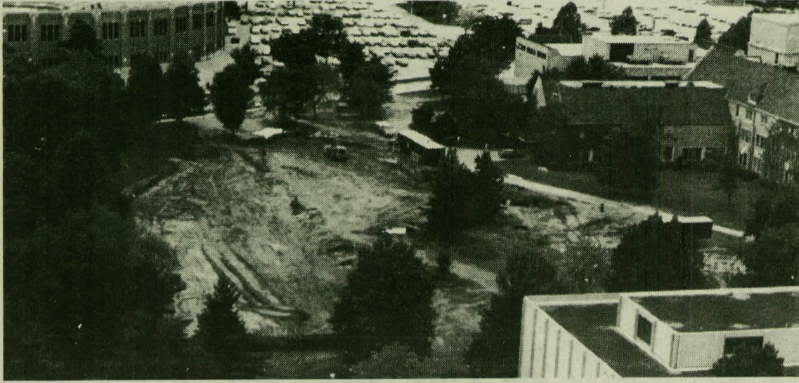
The sight of the new faculty office building is seen from the top of the Memorial Library. Clearing for the project, behind O'Shaughnessy Hall,
